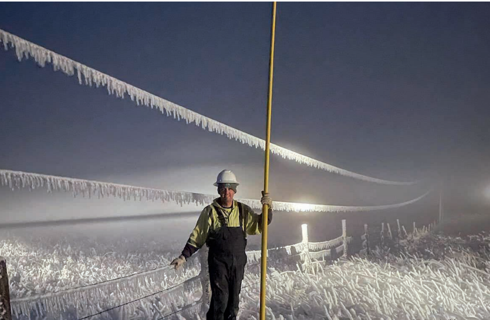
Journeyman Electrician Vinson Dargatz stands next to lines sagging from ice-build-up.
